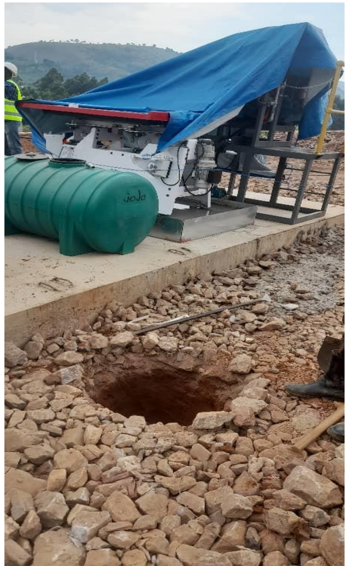
Earthing works in progress
