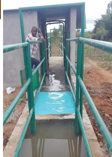
CONSTRUCTION OF SPRAY RACES
