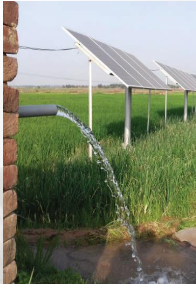
SOLAR WATER PUMPING
