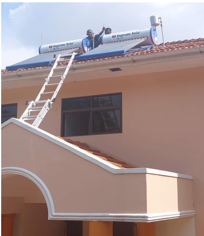
Solar water heater installation
