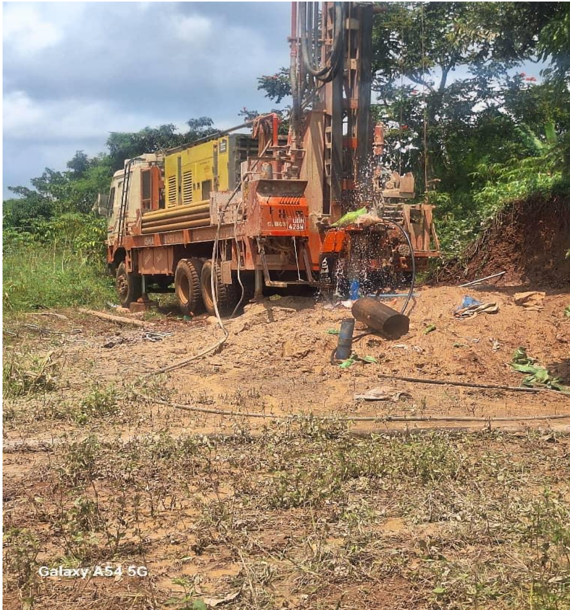
Borehole drilling works at Bbira COU SSS Ltd in Mukono, Bulimu.
