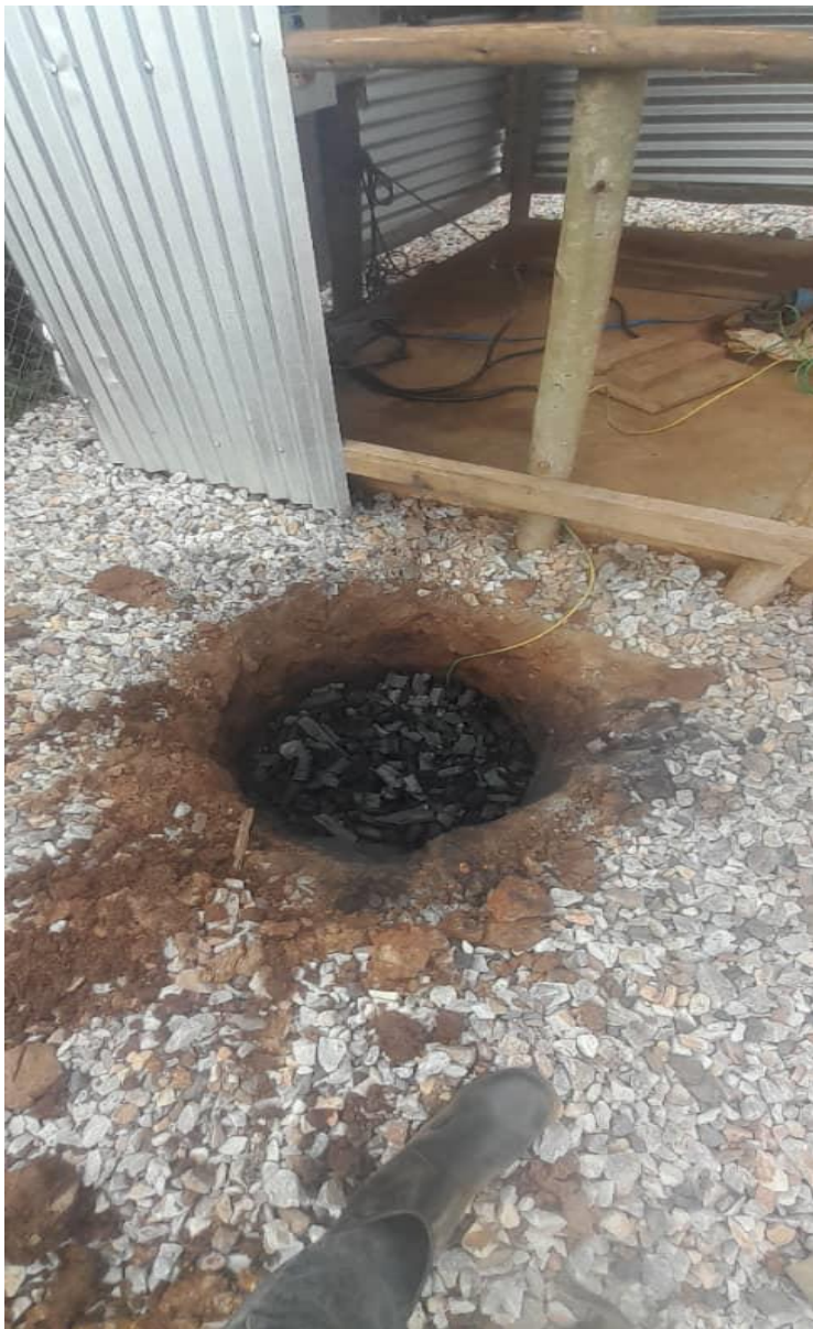
Earthing works in progress
