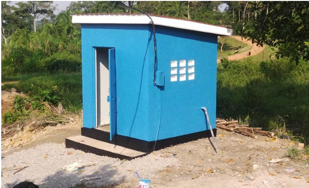
Completed construction of Pump house
